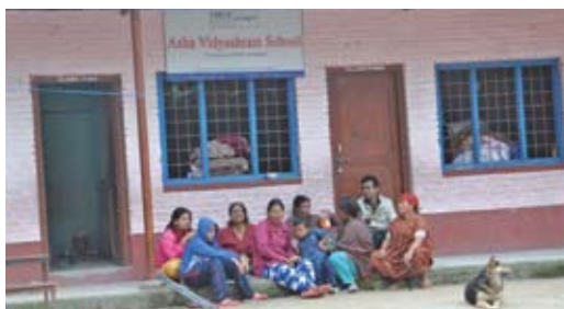
HOPE worldwide Nepal's school quickly became an emergency shelter after the earthquake.
